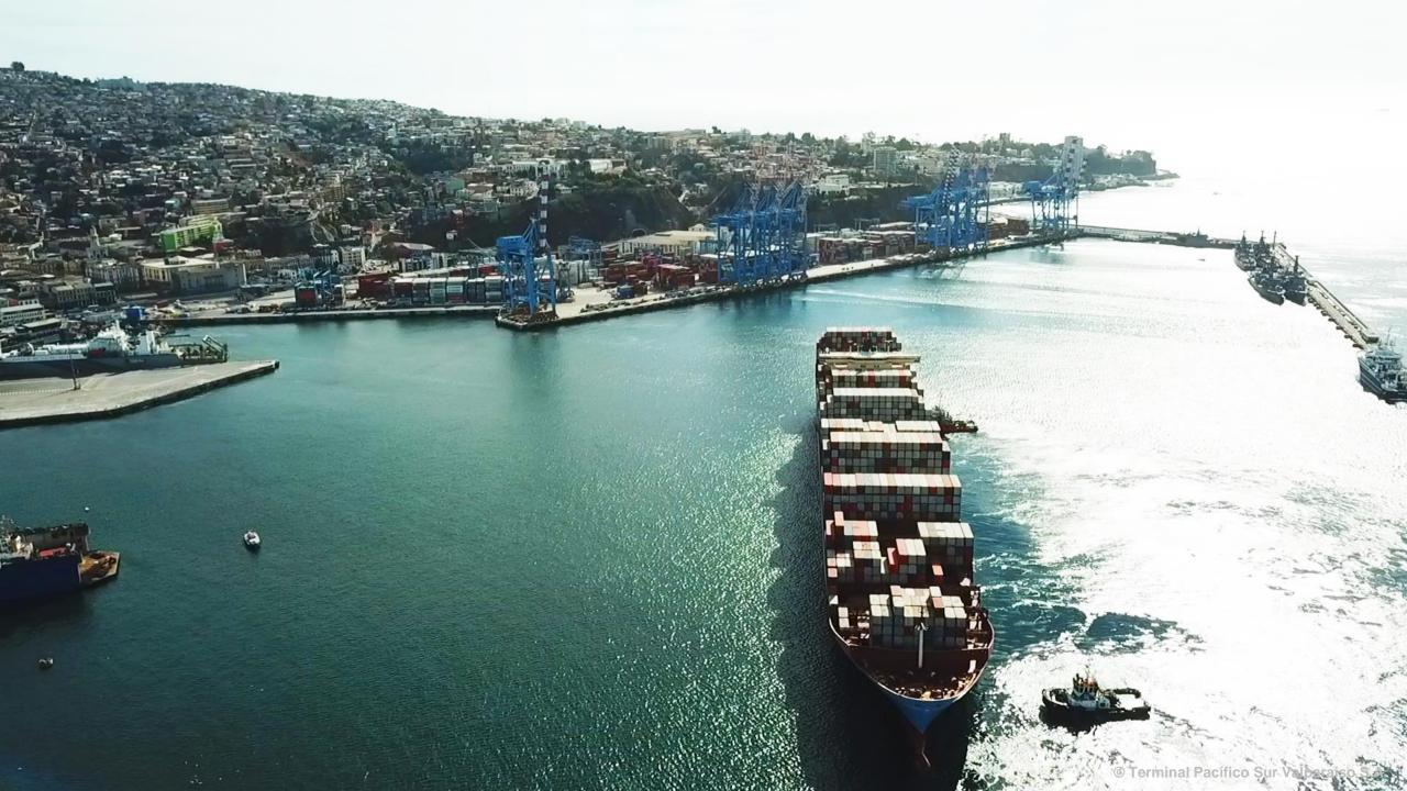
**OUR TERMINAL** Berthing quay and operational area **QUAY 1** QUAY 2 Design Vessel **Design Vessel LOA** 185m LOA 336m + LOA 336m 740m LOA 366m + LOA 300m 266m Max Draft 9.4m Max Draft 14.1m Operational area: 15ha
